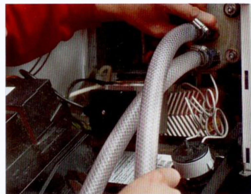
▲ Attaching flushing hoses to the power flush adaptor
