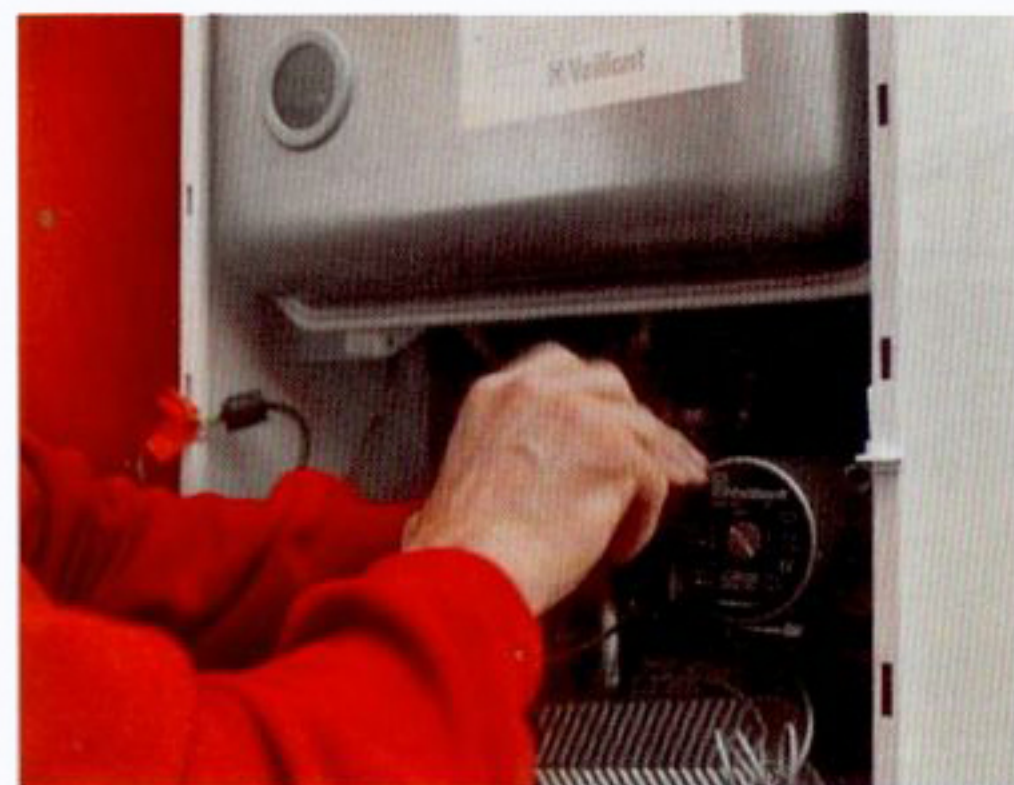
▲ Removing a boiler system's pump face
