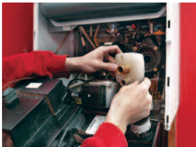
Photo 2. Attaching pump adaptor.
