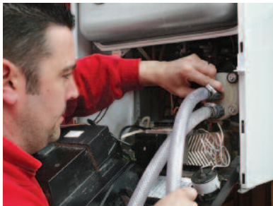
Photo 3. Attaching power flushing hoses.
