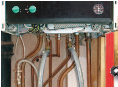
Photo 4. Combi boiler being descaled.
