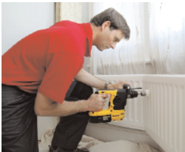
During powerflushing, radiators should be vibrated to remove debris build up
