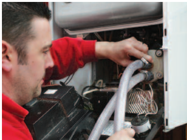
Photo 3. Attaching power flushing hoses.
