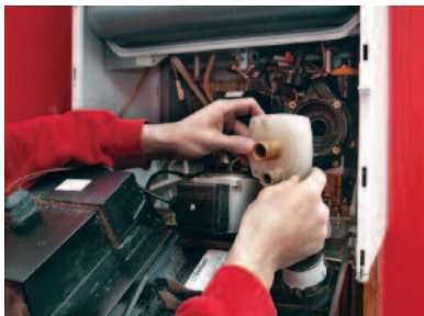
Photo 2. Attaching pump adaptor.
